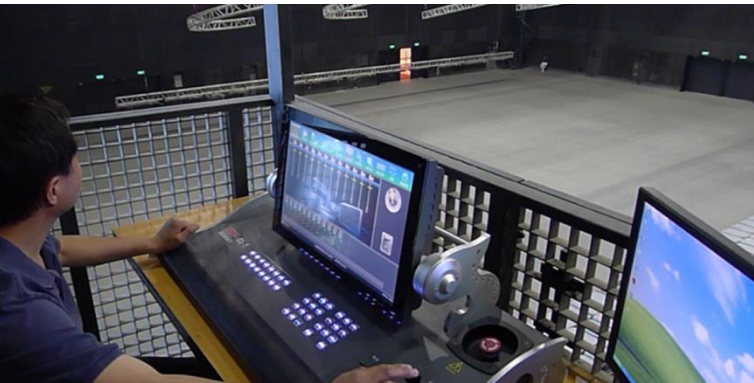
Lighting hoists are controlled by an intuitive hoisting controller.
