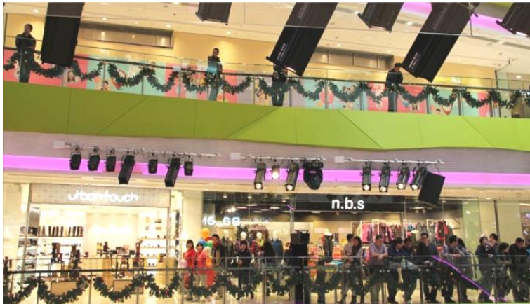
Over 50 Fresnel and Profile spotlights were installed.
