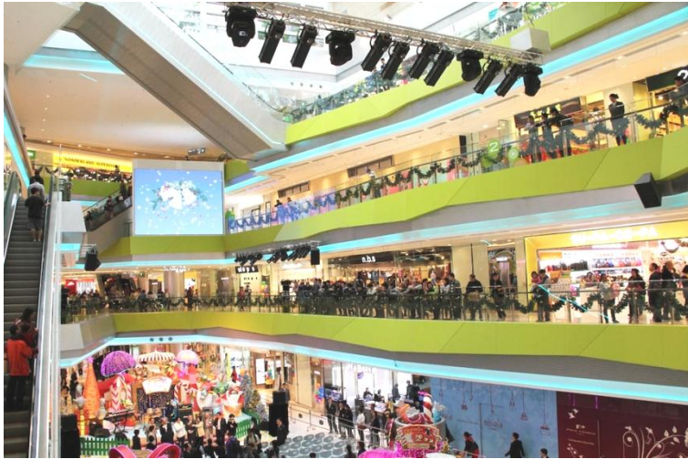
Lighting fixtures at L4 Atrium.
