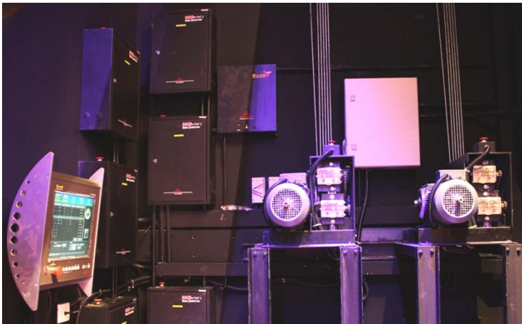
All Lighting bars are motorized and can be managed backstage by a touch-screen Hoist Controller.
