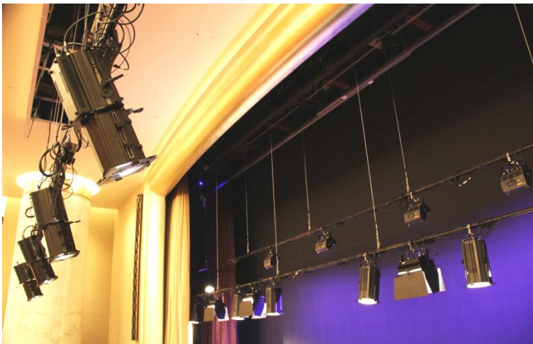
MacoLEDs LED Profile spotlights can be stored inside an automated ceiling cover system.
