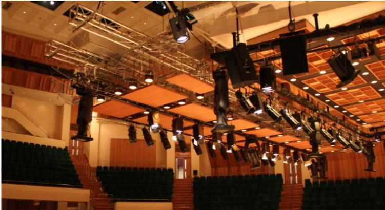
The extension of stage lighting system, installed with 70 downlights and profile spotlights with different field angles, can be raised and lowered above the stage, to provide better sound reflection for concert performances.
