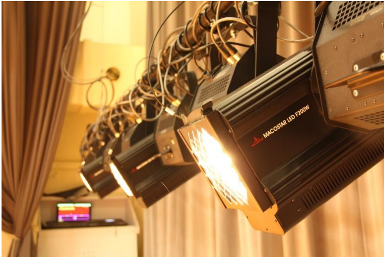
An energy-saving LED spotlight gives just as powerful output, but consumes up to 70% less electricity.
