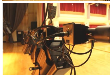
Rigging: Lighting bars and curtains are motorized and managed by a hoist control system. (left) Dimming: Stage lighting and house lighting fixtures are all dimmable. (right top) Easy routing: DMX ports on lighting bars for easy and direct connection to DMX devices. (right bottom)
