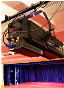
Users can access the LED Profiles from the side stage Lighting Tower (left), and easily adjust light beams with their built-in shutters.
