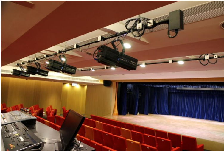
These cool white LED profiles not only give powerful light beams simulating natural daylight, but also have RDM built inside, ready for remote setup of DMX addresses for dimming and other functions.
