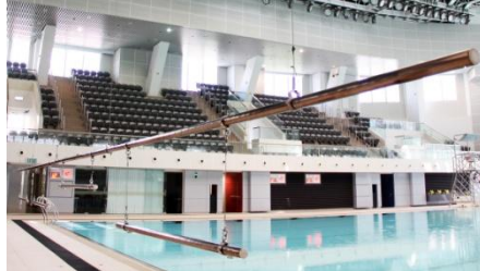
Flag raising bars are attached to the steel wires (bottom right) which pass through the rigging blocks up at the ceiling's fly system (left), then back to a variable speed flag raising drum winch (top right).
