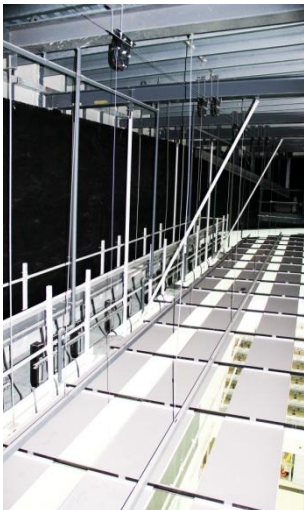
Flag raising bars are attached to the steel wires (bottom right) which pass through the rigging blocks up at the ceiling's fly system (left), then back to a variable speed flag raising drum winch (top right).
