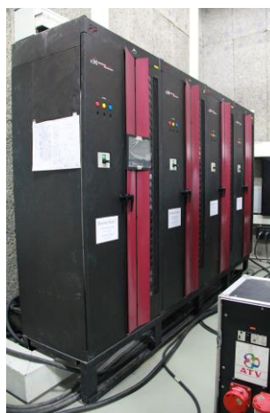
DPR Dimmers are equipped for the 1900 m 2 Studio 8, ATV's largest production studio.
